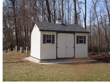
Outdoor Utility Shed
